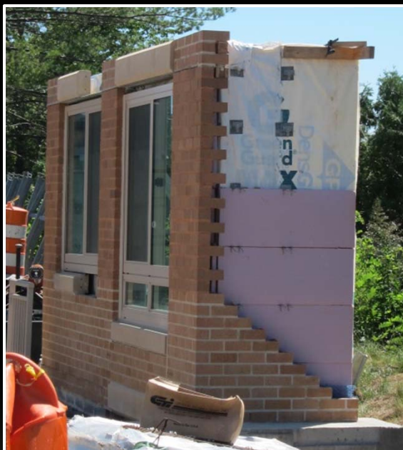
IMAGE COURTESY OF HITT CONTRACTING
