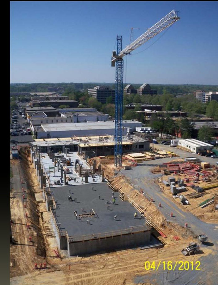
IMAGE COURTESY OF HITT CONTRACTING
